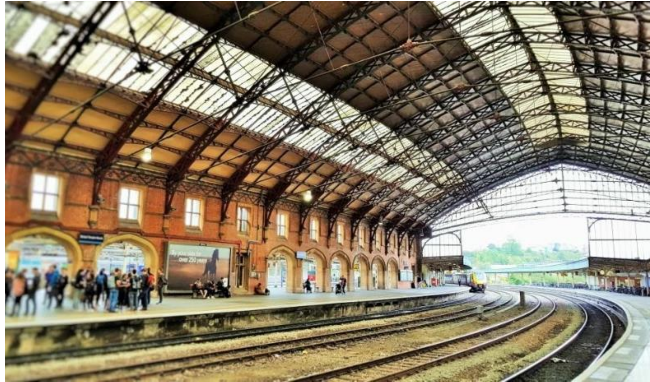
Temple Meads Roof, Bristol. 125 feet clear span 1876. (Grade I)
