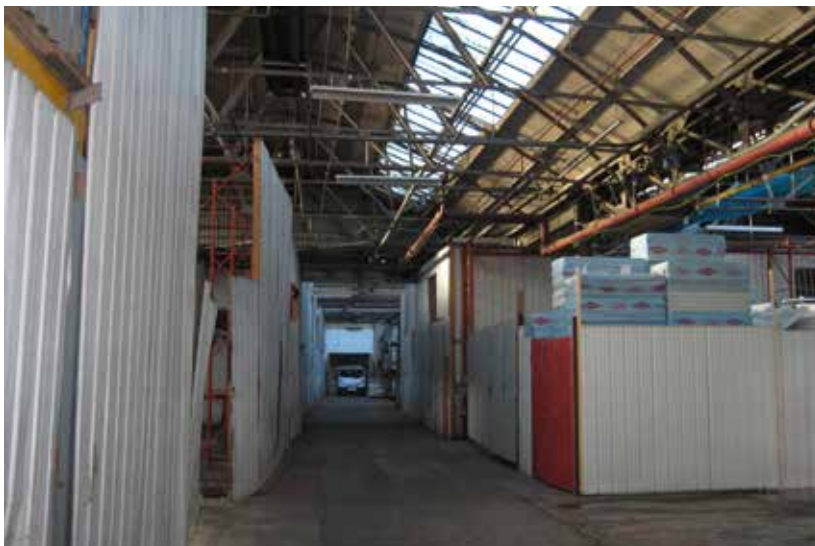
One of the bowstring truss roofs with inserted storage units and offices beneath
