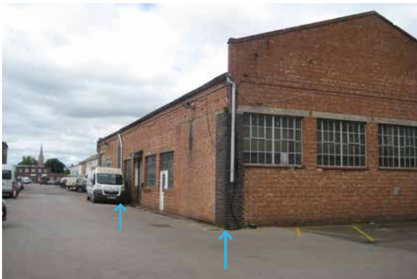
View south-westwards along the south-eastern elevation of Unit 1; the space between the two dark brick piers (marked) was historically openable, but has been infilled with brick
